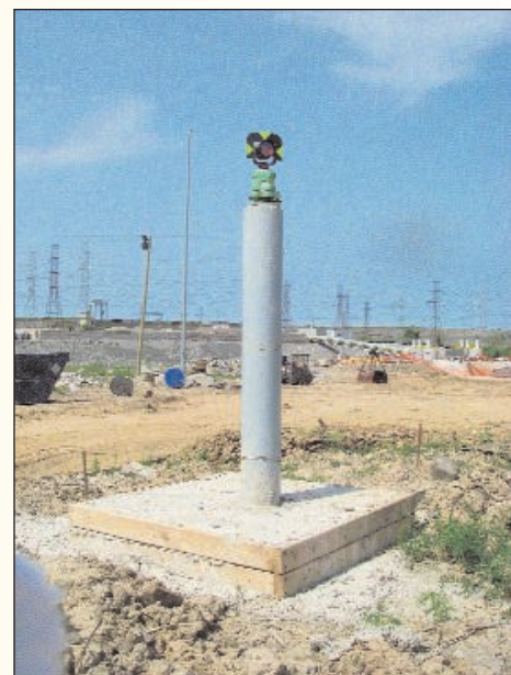
Figure 3.1.1 Pillar type of survey monument at Outlet area.
